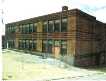
Rear of building with area that could provide 20 addl. spaces
