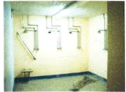
View of the shower area in one of the locker rooms
