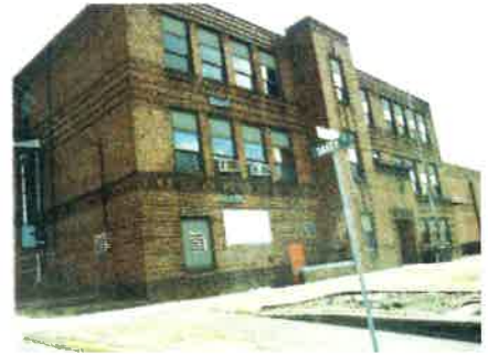
Another view of the front of the building
