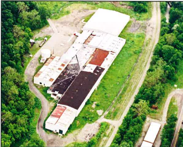
Colliers Steel, Colliers
