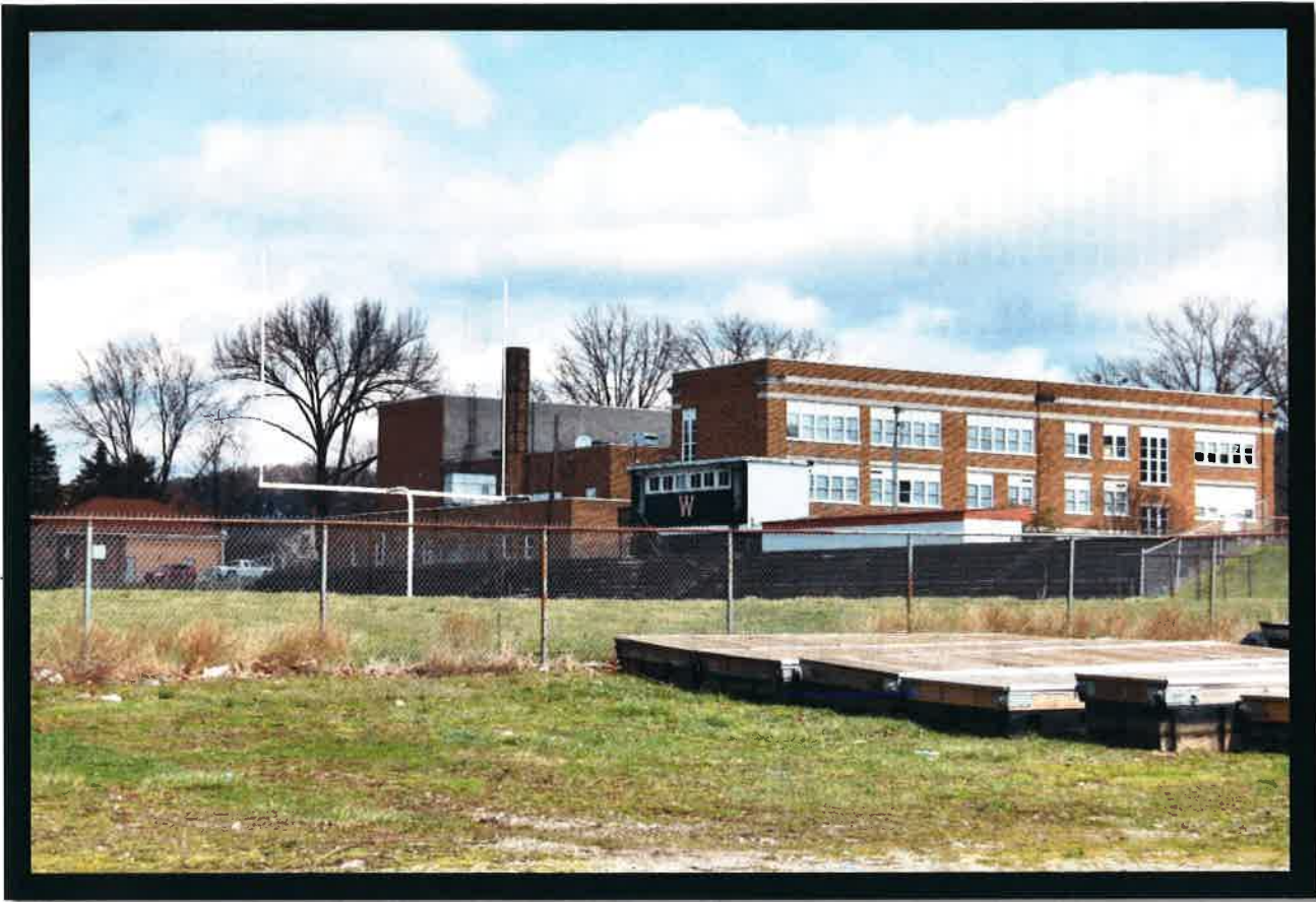
Southwest corner of the building
