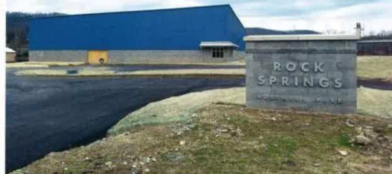
1 Rock Springs Business Park - Chester
