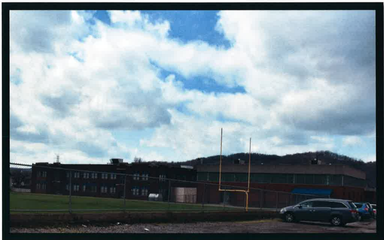
Back view of building and field house
