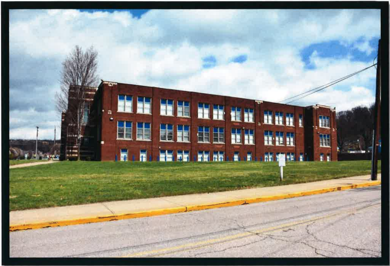
South side of the building
